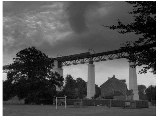
Spoorwegviaduct in Moresnet
